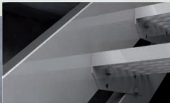
Supporting beam serves as a toe board
