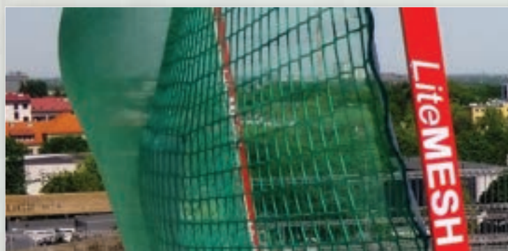
100x100 mesh catching falling objects, tools. Mosquito net catching small elements.
